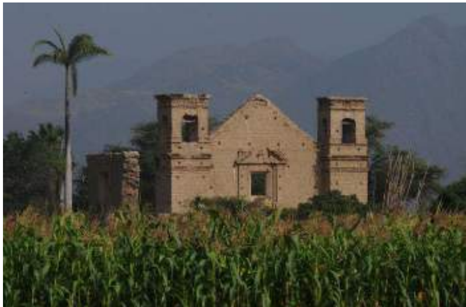
Façade of La Merced church: surrounded by vegetation.
