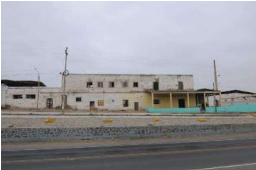
Present-day view of the former Úcupe hacienda, in the lower part of the Zaña Valley.
